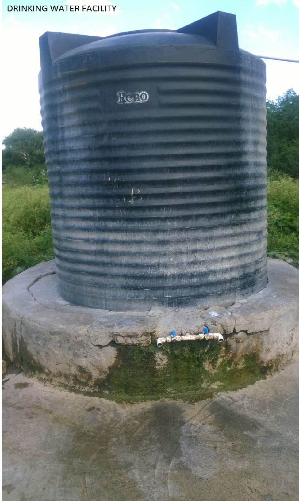
Drinking Water Facility
