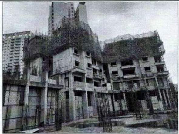
Fig: Construction work at the site
